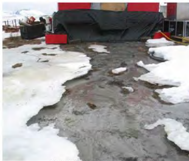
Figure 4. Water and cuttings discharge on uplands.
