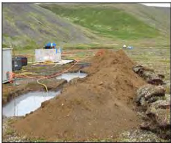
Figure 3. Sump pits (on left) and tundra stock pile being saved for reclamation (on right).
